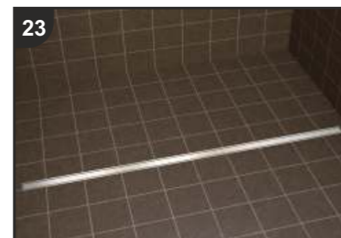
23 Griglia Double Face montata con la superficie in alluminio lucida in vista. In this view Double Face grid's polished aluminium side is mounted.
